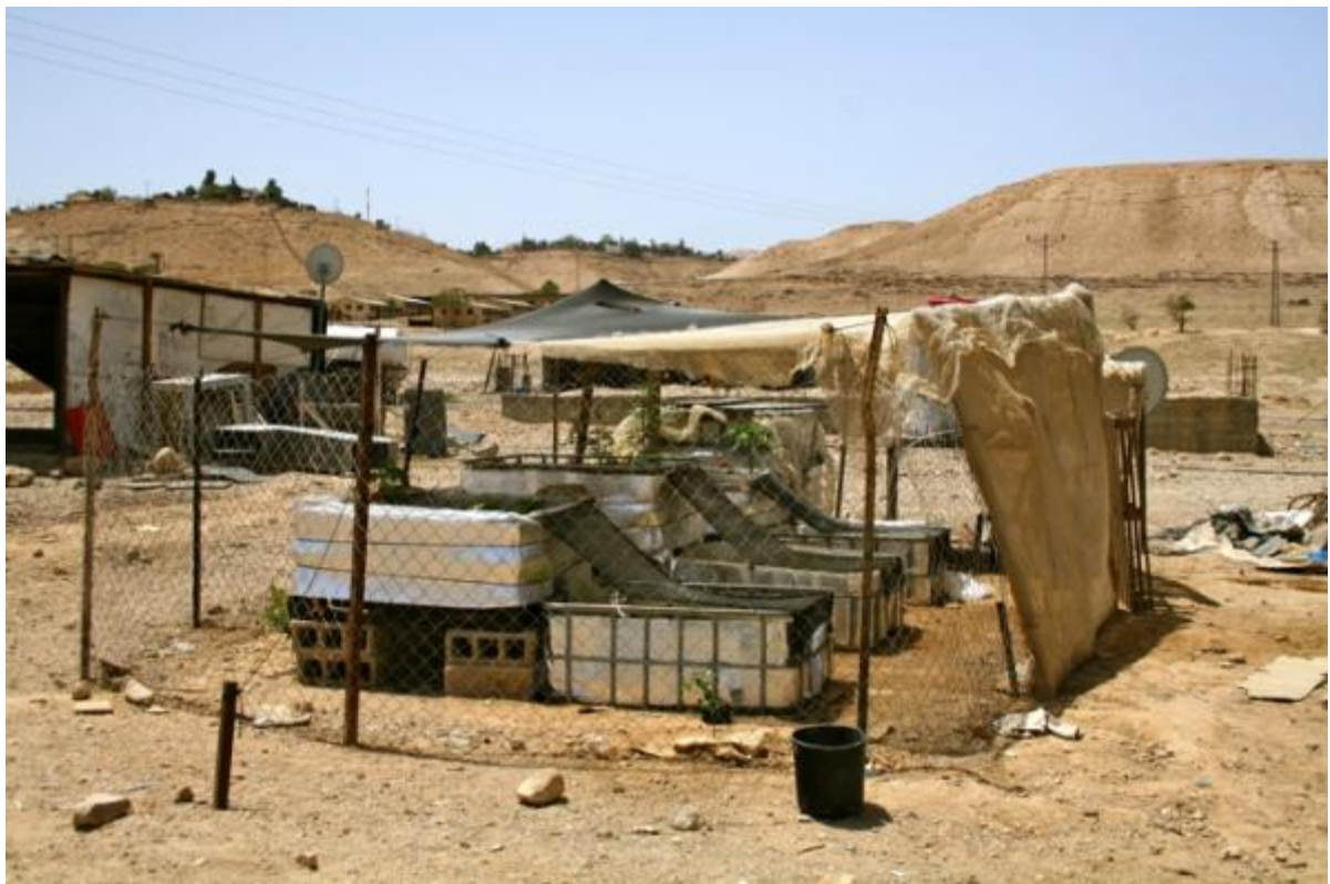
Figure 18: An operational aquaponic system. Note the fence and shade structure which could benefit from improvement.
