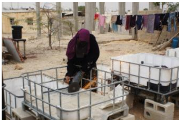
Figure 11: cutting a hole in the pallet to make space for the pipework
